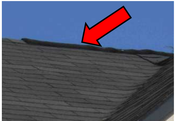
Ridge shingles missing (same area) Dark black area is plastic ridge vent
