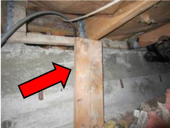
Joist supported with 2 x 8 non treated wood
