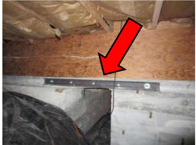
Foundation sections secured with metal connector
