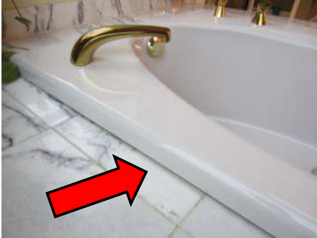
Tub should be caulked to tub deck
