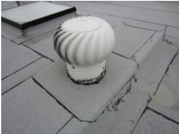
Roof vent (typical)
