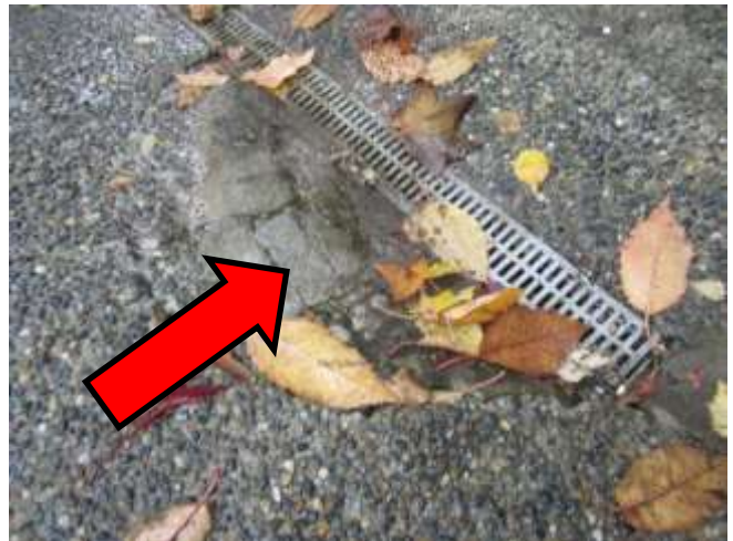
Concrete repair at driveway channel drain
