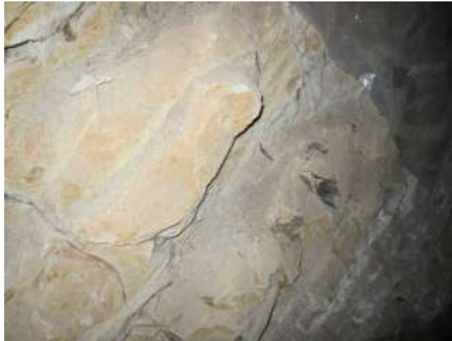
Bearing ground at Living room is rock; vertical cut of 6' +
