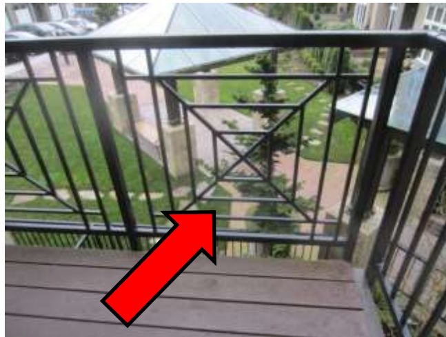
Ladder style barricade
