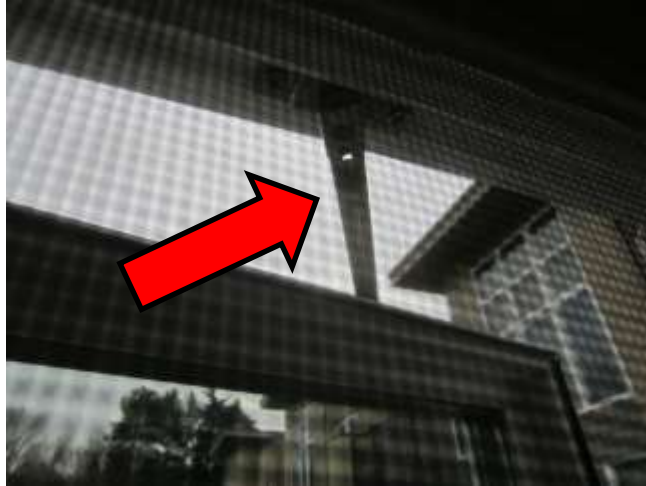
North window has limiter installed All others have been removed
