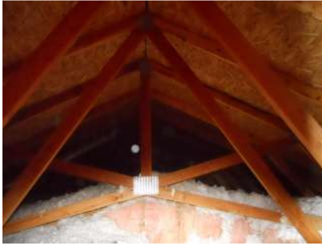
Vaulted ceiling above Living room and Kitchen
