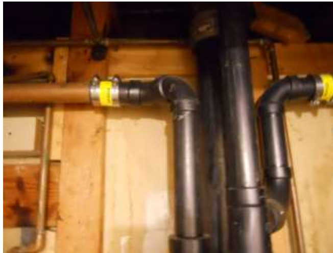
Prior repair to plumbing pipes in Utility room area
