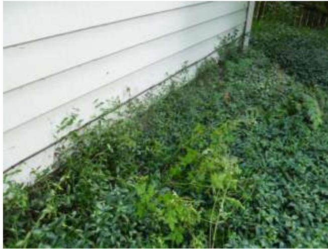
Vegetation should not be in contact with the house (including the roof)
