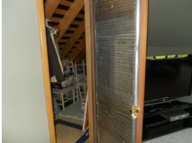
Closet door is not weather rated
