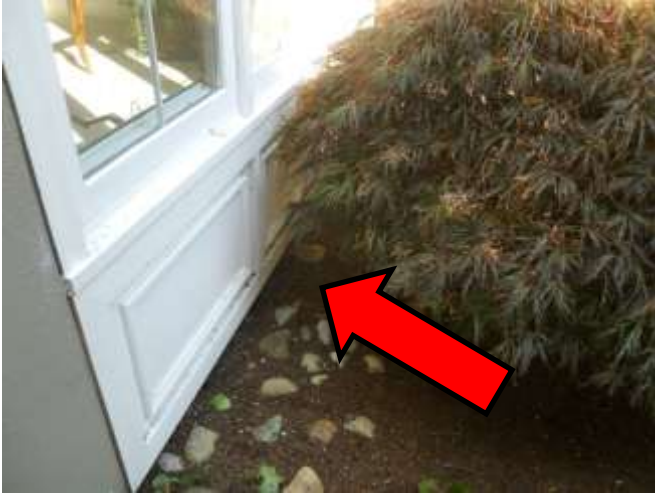
Earth to wood contact (typical)
