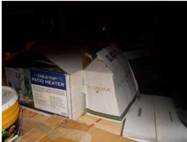
Wood and cardboard should not be stored in crawlspace
