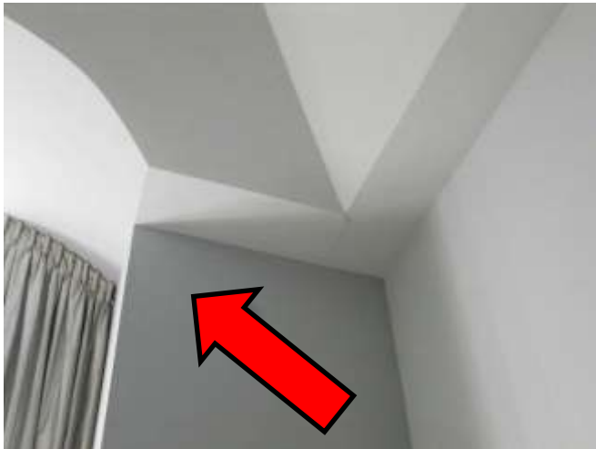
Moisture stains on wall
