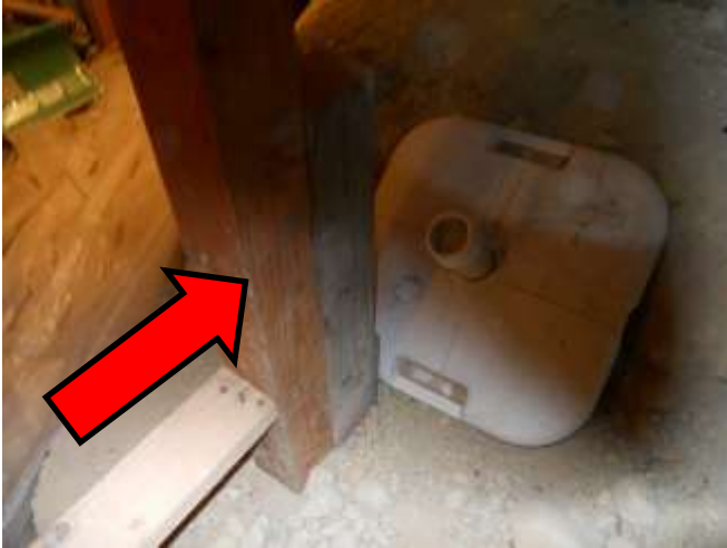
It appears a new post was installed
