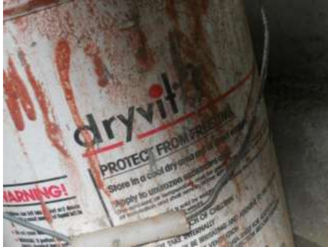
Empty bucket of “dryvit” in crawlspace
