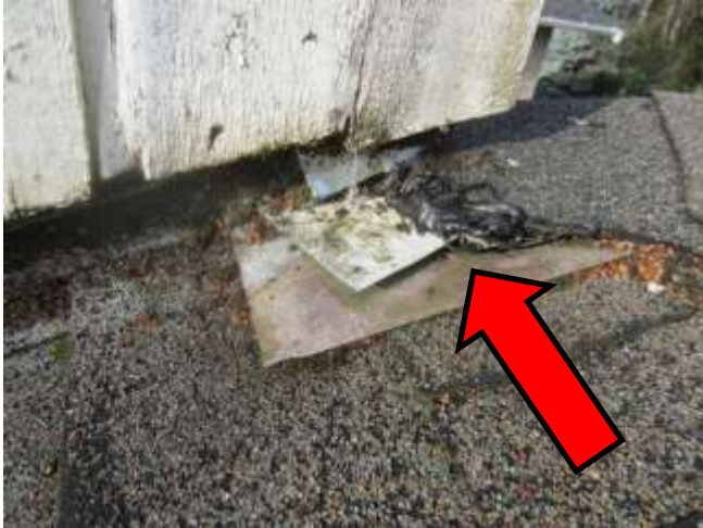
Tar has been spread at the upper corner of the chimney
