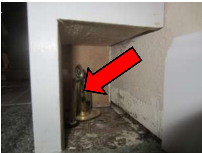
Unable to quickly rotate gas valve key
