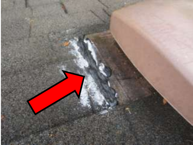
Tar repair at Hat vent
