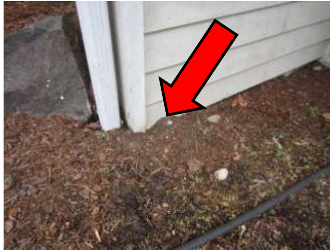
Earth to wood contact (typical)
