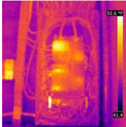
No evidence of over heating
