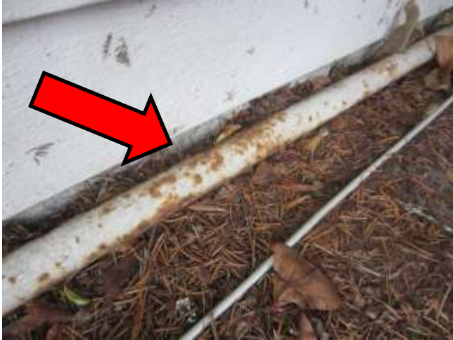
Gas pipe lying on the ground
