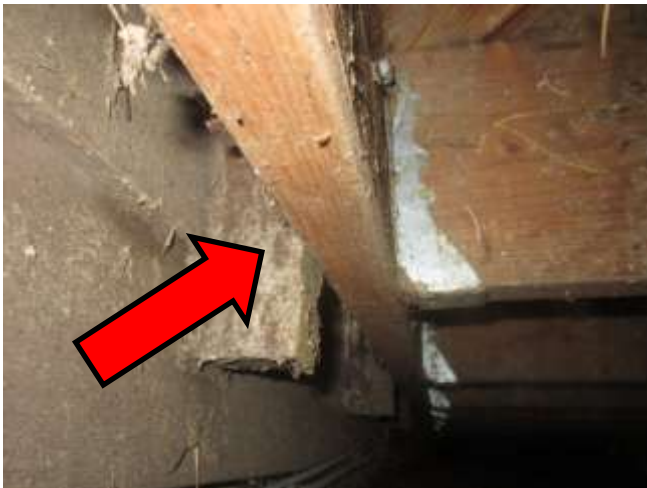
Connection to cut cantilevered joists
