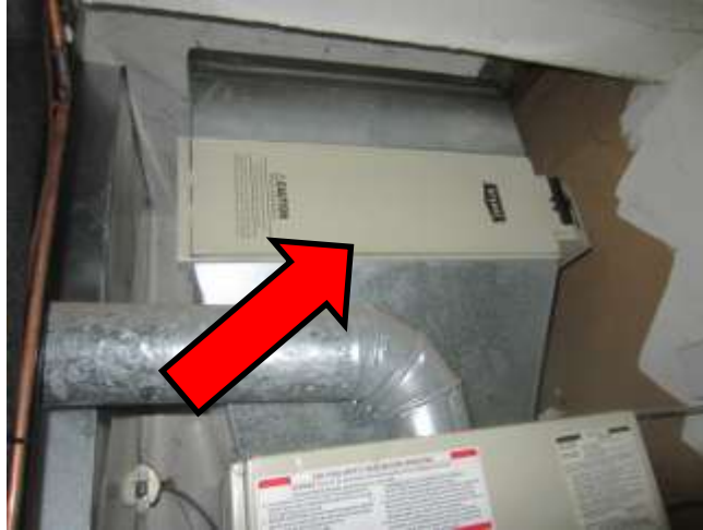
Furnace filter location
