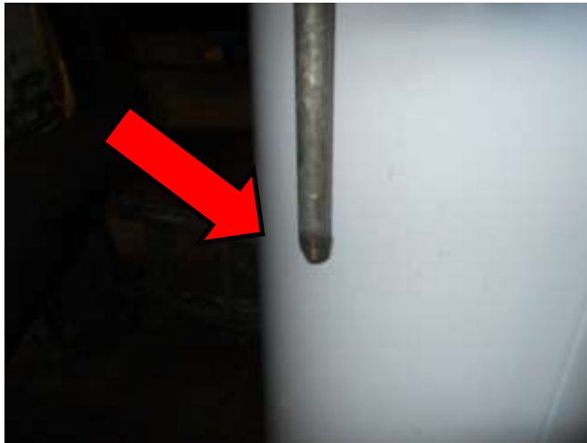
TMP line should not be threaded at end
