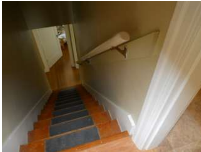
Steep stairwell with wood treads
