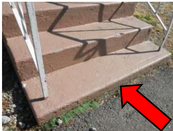
First step height is not consistent with other steps
