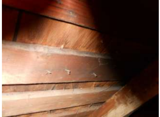
Shake roof on skip sheathing
