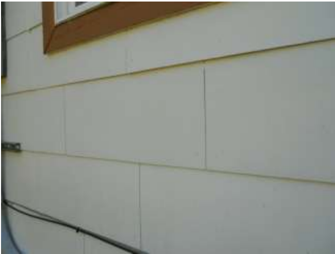
Siding appears to be asbestos type
