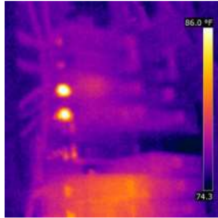
No evidence of over heating
