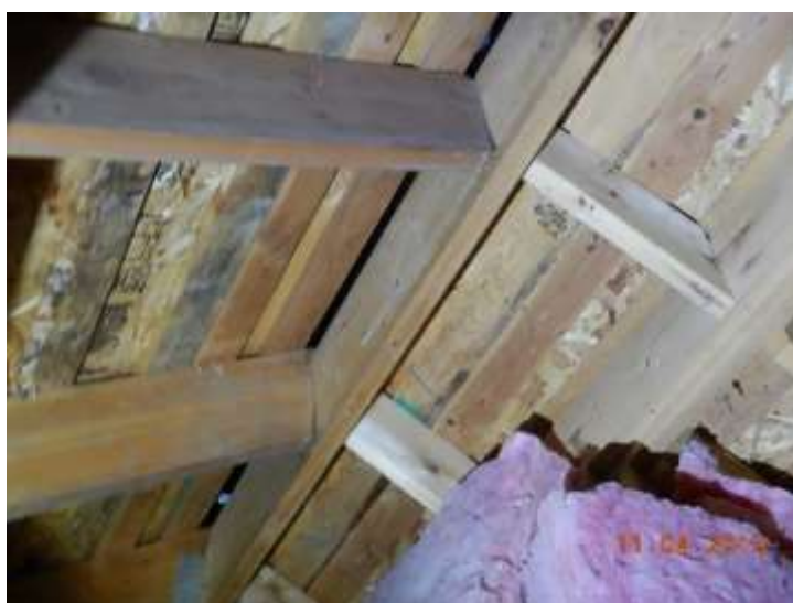
Roof framing/ venting
