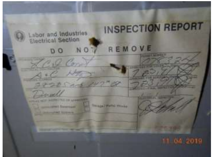
Electric service permit tag
