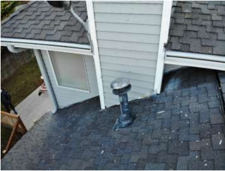
Garage area roof
