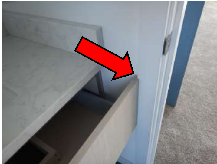
Drawer strikes the door casing
