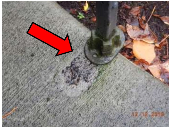
Unsecured handrail
