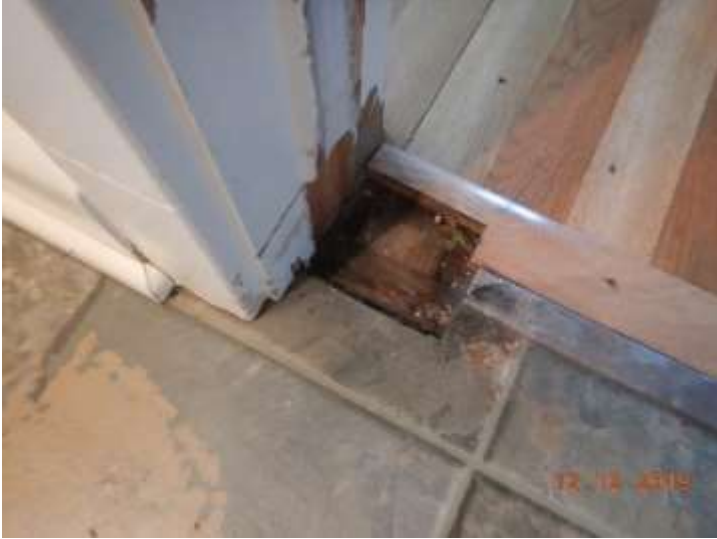
The door to the Dining room has been removed
