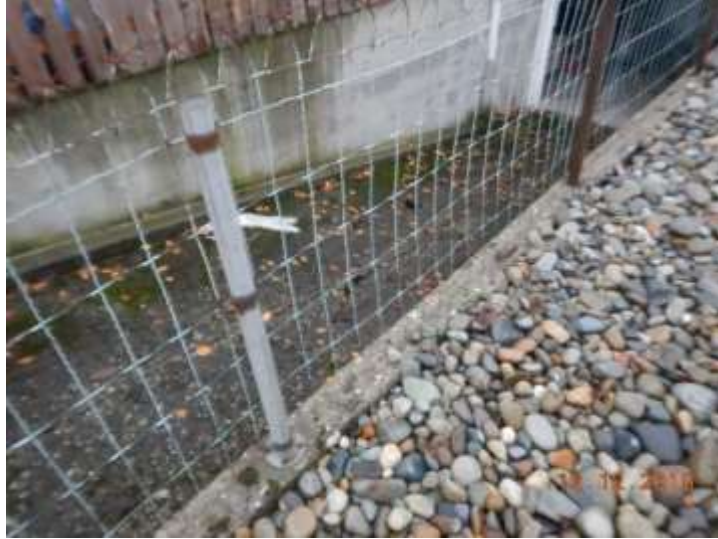
A safety barricade is installed at the upper side of the driveway
