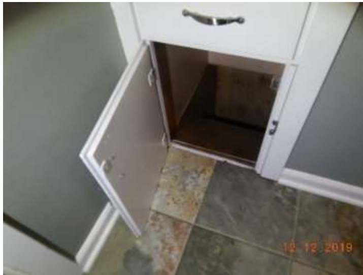
Laundry chute at floor level
